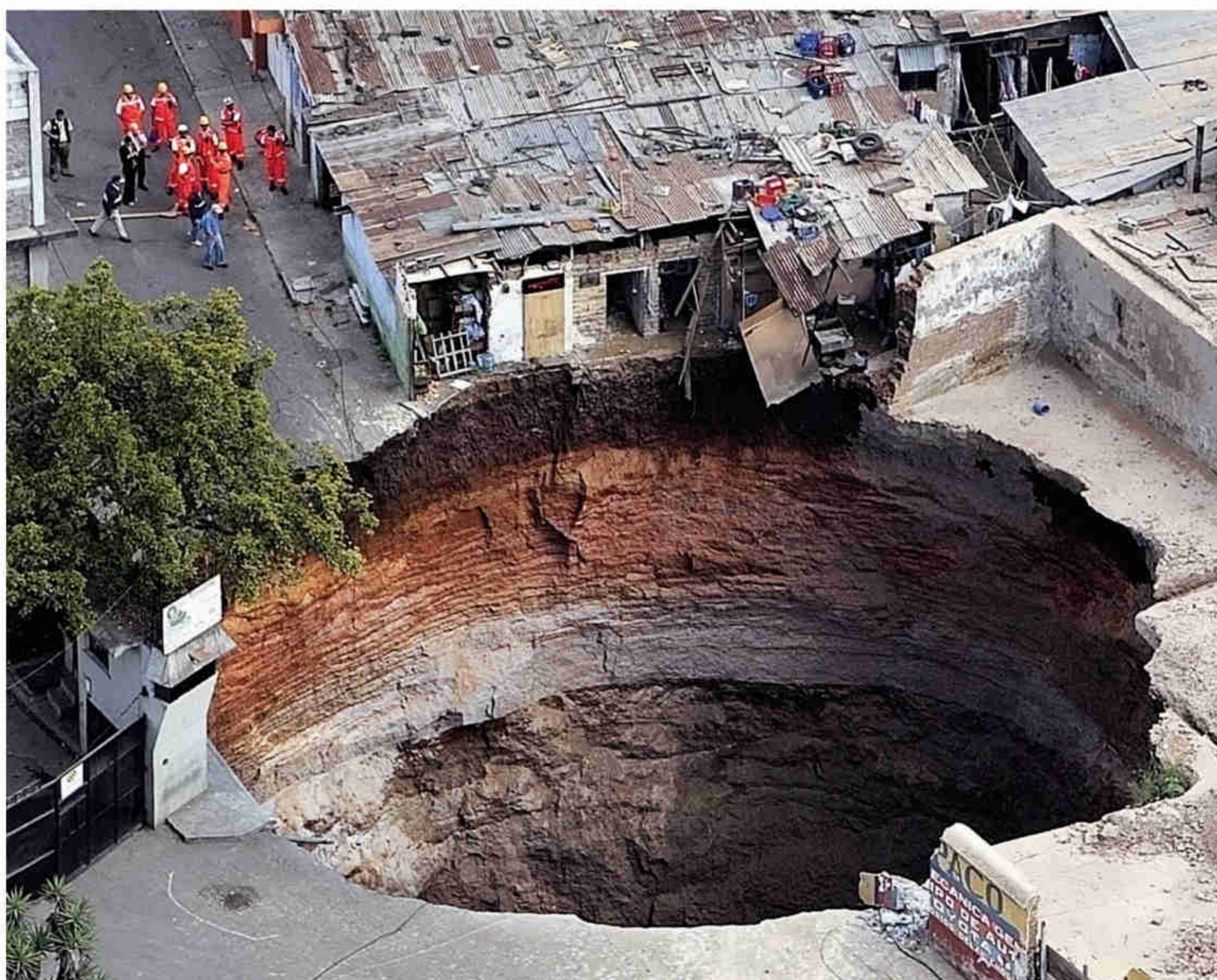
In 2007, a giant sinkhole in Guatemala City claimed three lives and swallowed several houses.
